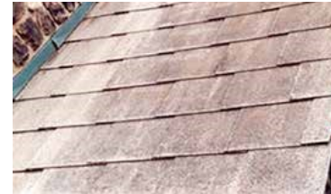
Asbestos cement shingles
