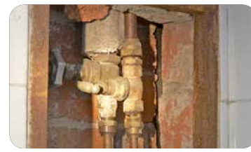
Friable asbestos lagging on pipes
