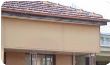
Asbestos cement sheeting in eaves
