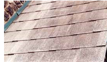
Asbestos cement shingles
