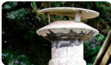
Asbestos cement flue and cowl
