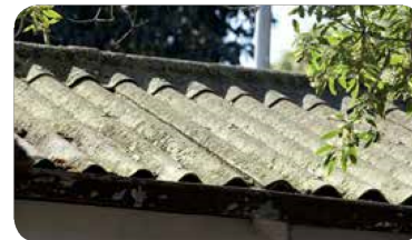
Asbestos cement corrugated roofing
