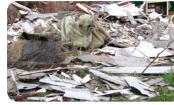
Broken asbestos cement materials from a demolition
