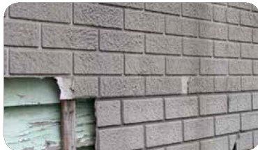
Asbestos cement 'brick' cladding
