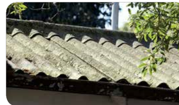
Asbestos cement corrugated roofing
