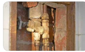
Friable asbestos lagging on pipes
