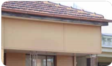
Asbestos cement sheeting in eaves
