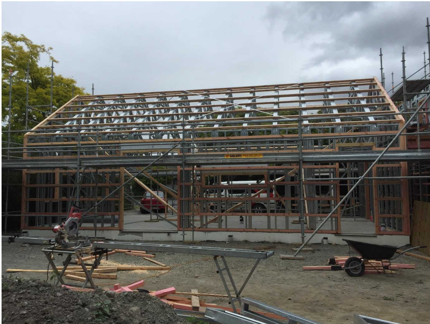
Steel framed living pavilion , fast construction of frame
