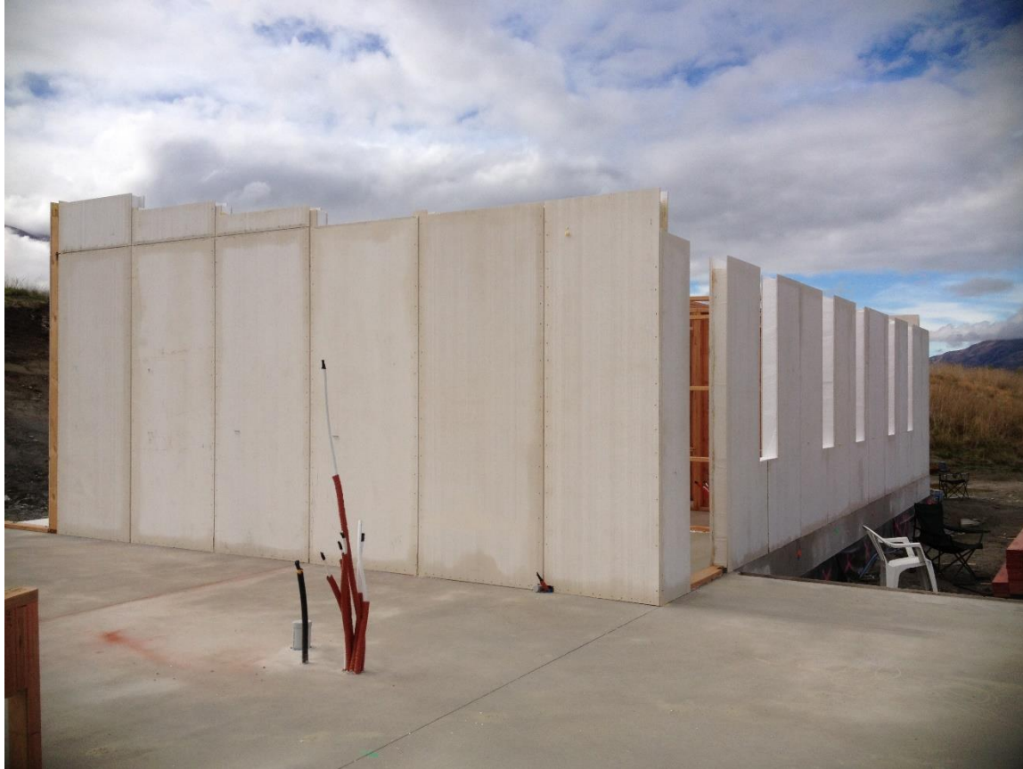
MagRoc panels being installed
