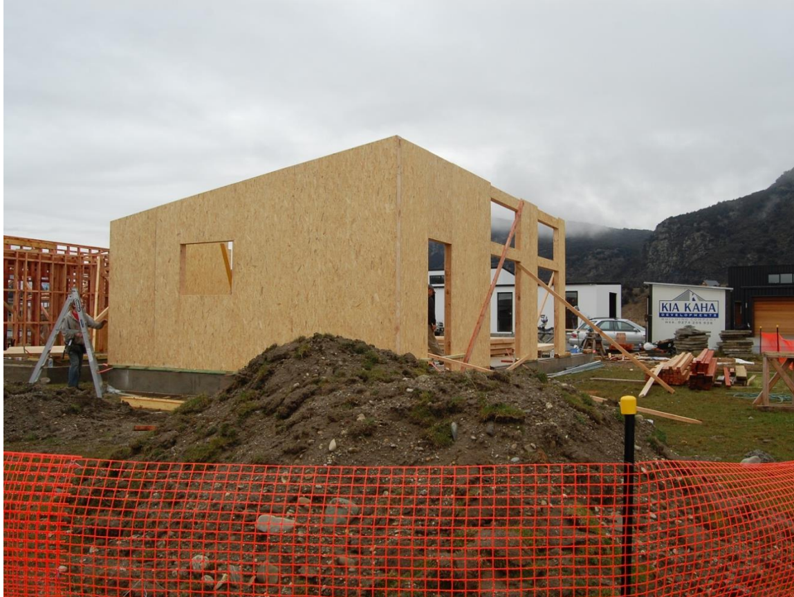
First pavilion under construction
