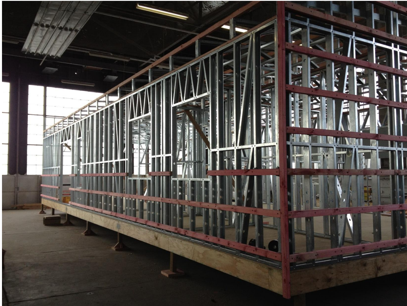
Steel framed house constructed off site
