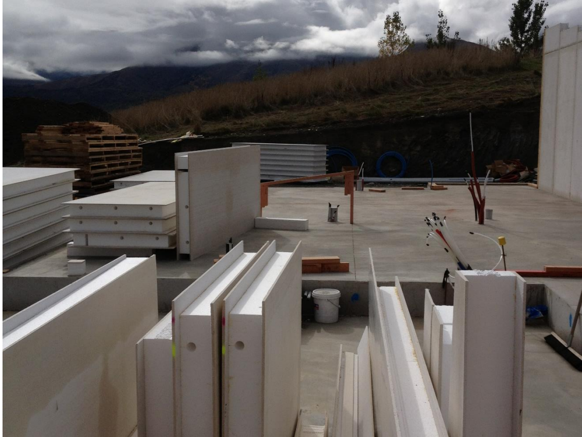
Magnesium oxide panels with polystyrene core and conduits for services
