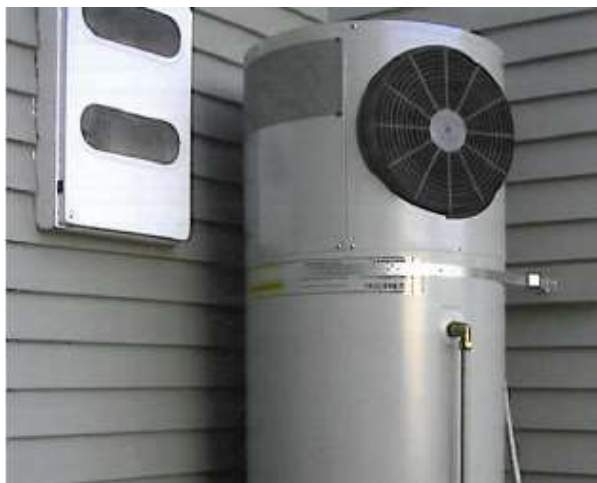
An integral heat pump hot water cylinder is usually sited outside. Photo: BRANZ Bulletin 529 Dec 2010
