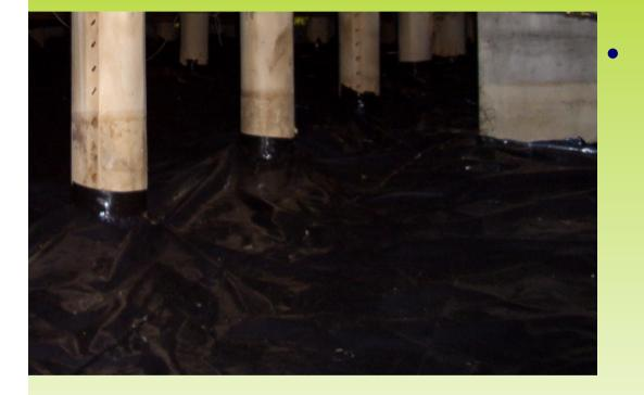
Installing a damp proof membrane on the ground under your floor stops up to 40 litres of moisture coming up from under your home each day
